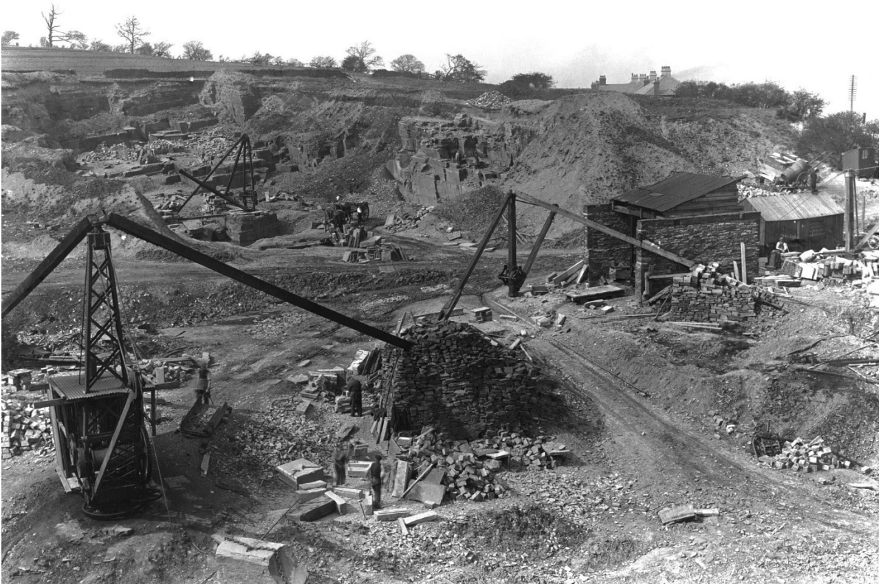
Figure 7. Photograph P201122 – Former Flagstone Quarry in the Greenmoor Rock, Meadowhead, Sheffield, looking NW. The site is now occupied by Morrisons supermarket. From British Geological Survey Geoscenic imagebase, Photograph P201122 , date May 1911, reproduced by courtesy of the British Geological Survey (N.B. the image in Geoscenic is reversed).
