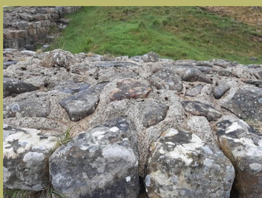
Section of the wall showing infill and lime mortar
