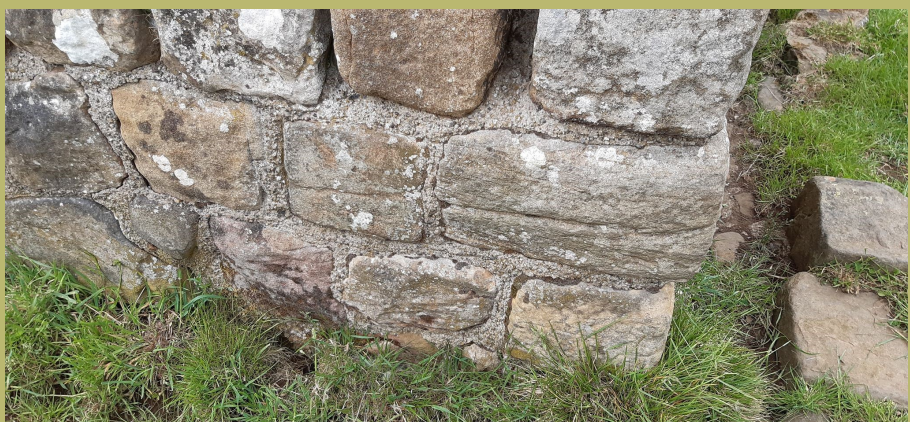
Section of the wall at Milecastle 39 showing outer sandstone blocks and lime mortar
