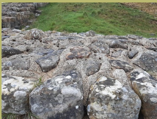
Section of the wall showing infill and lime mortar
